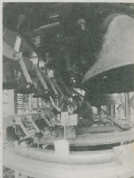
Installation work in progress on the Bournville Carillon
