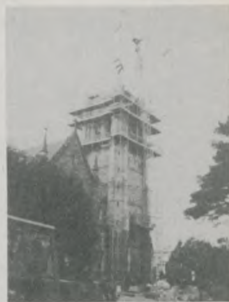
Frame side being lowered into St. Saviour's Cathedral, Goulburn, N.S.W., Australia
